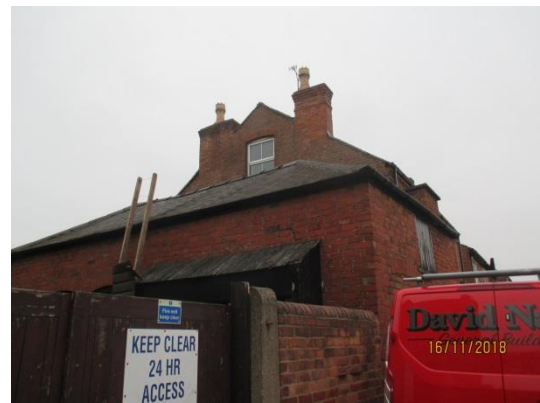
Second floor window in 1 Mona St with on-site outbuilding below
