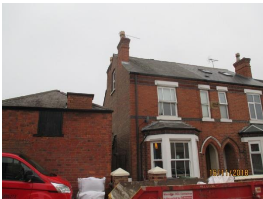
1 Mona Street, adjacent to outbuilding
